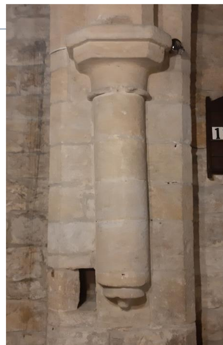
One of the four Norman corbels at the corners of the Nave.
