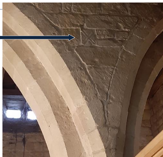
The St Andrew's Cross visible from the North wall by the Kitchen
